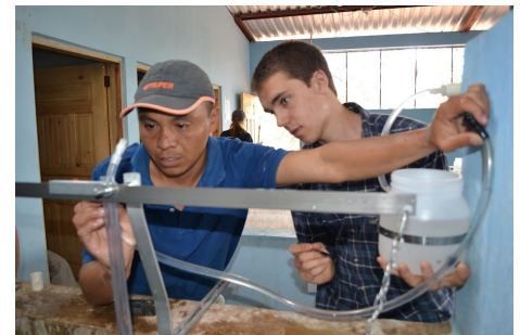
AguaClara's chemical dosing technology to disinfect water supplies was installed in 18 villages in India in 2013.
